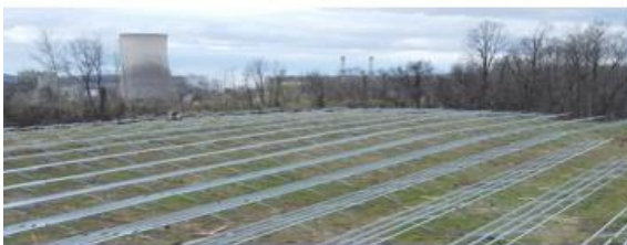
Foul Rift - 19 MW Under Construction
